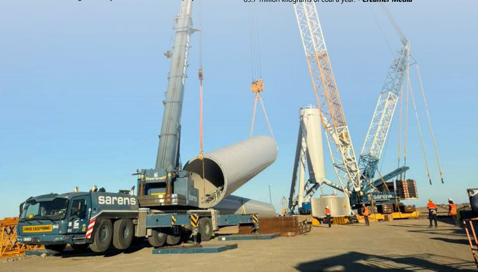
INSTALLATION: A Sarens Siba crane lifting heavy equipment at the site of the InnoVent Diaz onshore wind farm.
