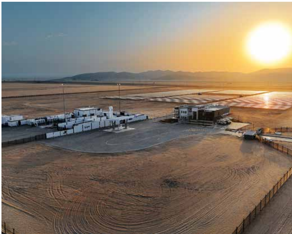
GREEN ENERGY: The Cleanergy facility uses solar energy and battery storage to produce hydrogen through electrolysis, and includes storage tanks, a mobile refueller, and Namibia's first hydrogen academy.
