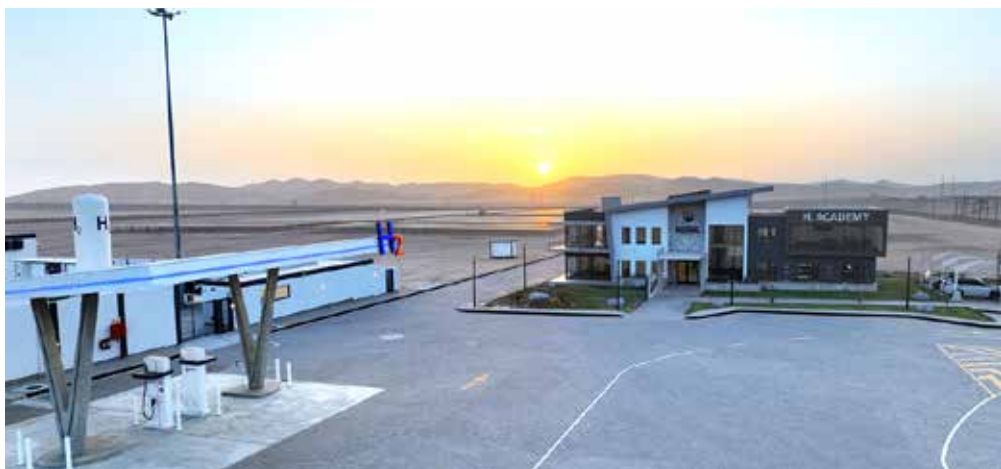
GREEN ENERGY: The Cleanergy facility uses solar energy and battery storage to produce hydrogen through electrolysis, and includes storage tanks, a mobile refueller, and Namibia's first hydrogen academy.
