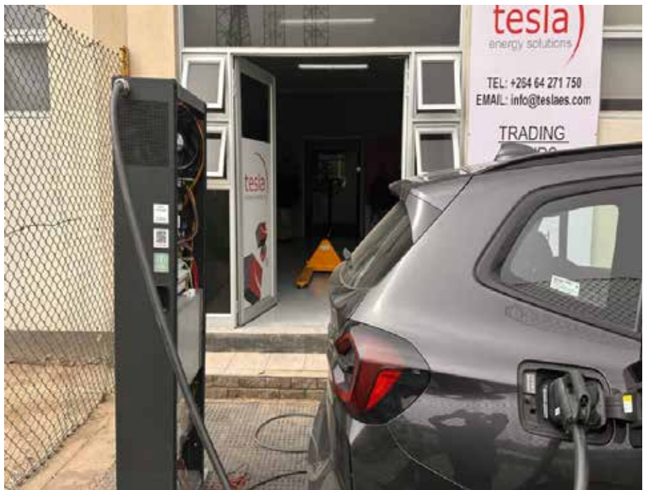
QUICK CHARGE: Testing of a 80 KW fast DC charger.
