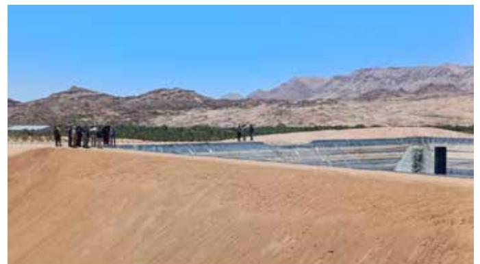
SOLAR-POWERED: 18 000 m 3 dams constructed by Brandberg Construction and powered by 100% solar energy.
