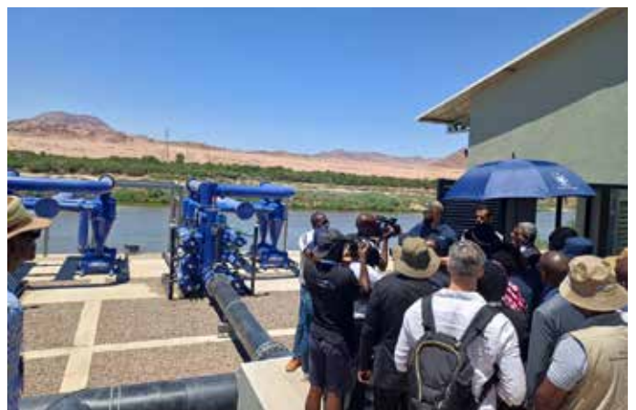
NEW STATION: Inauguration of the river extraction pump station.
