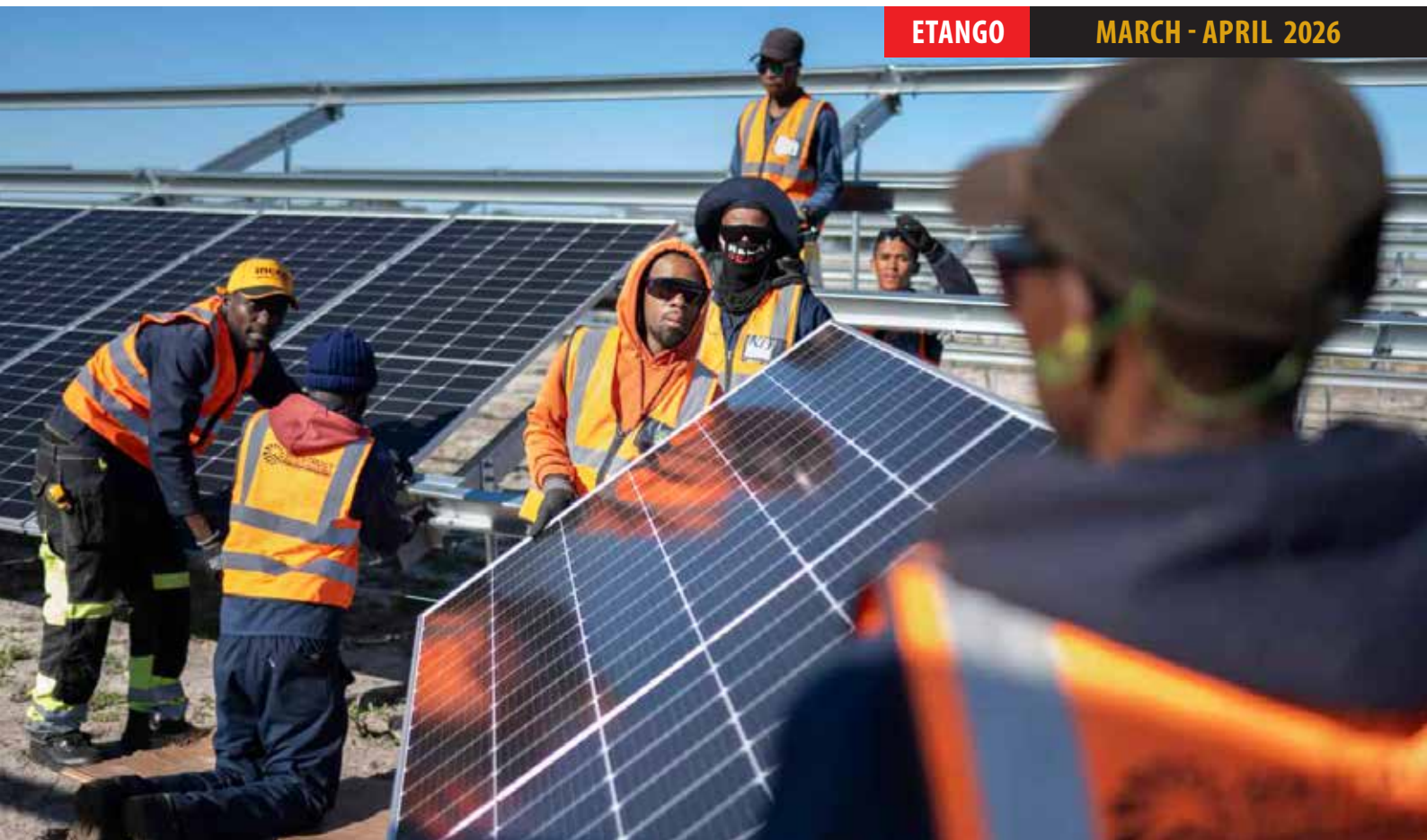
SUN POWER: Workers fit solar panels onto frames at South Africa's first municipally owned solar plant, June 5, 2025, in Atlantis, about 40km from Cape Town.
