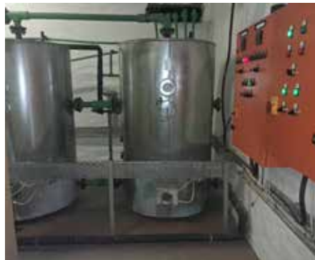
REVAMP: The Maternity Ward received a revamp to the existing boiler system including pump replacements and control board repairs
