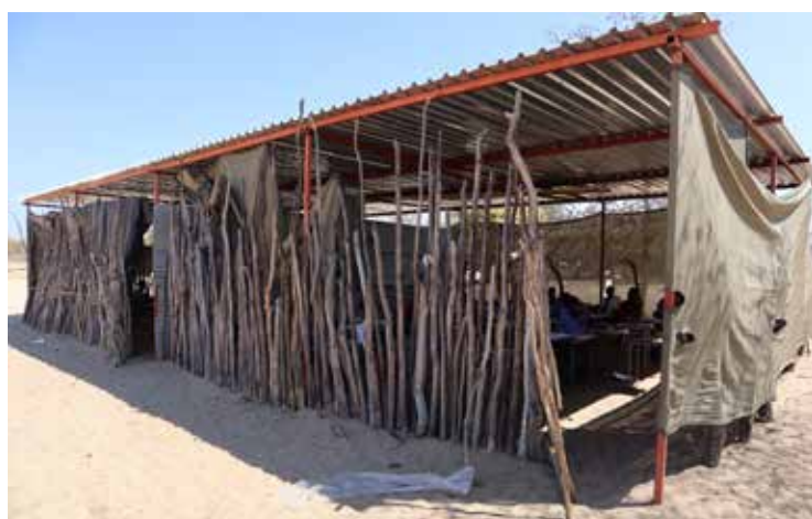
HARSH CONDITIONS ... Two temporary classrooms constructed by community members to help address the shortage of classrooms at Omatope Primary School in Oshikoto Region.
