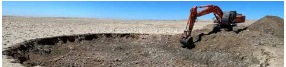
DIGGING DEEP: Foundation works at Diaz Wind Farm. Photos: InnoVent
