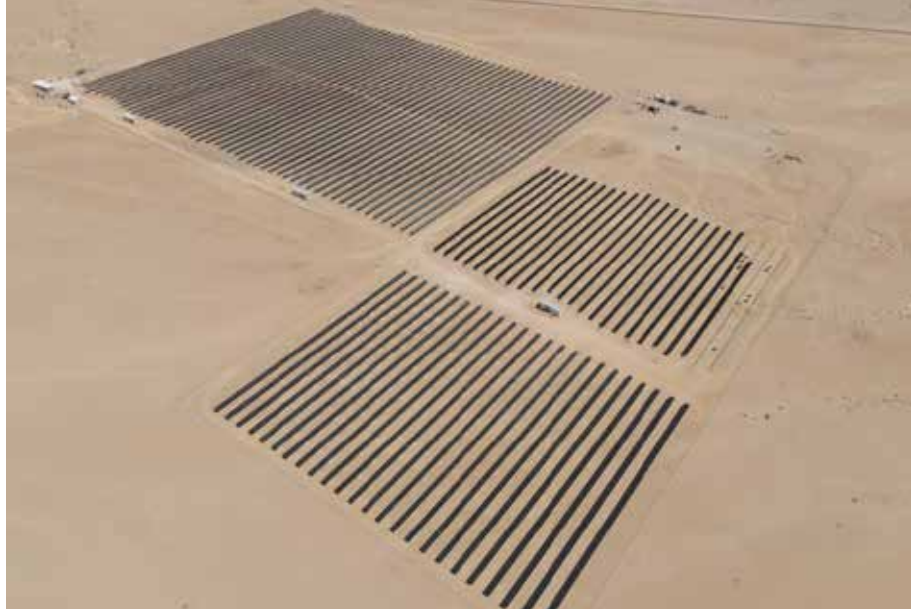
INNOSUN'S 5th SOLAR PARK: The Sorexa solar project near Arandis under construction. Photo: InnoSun
