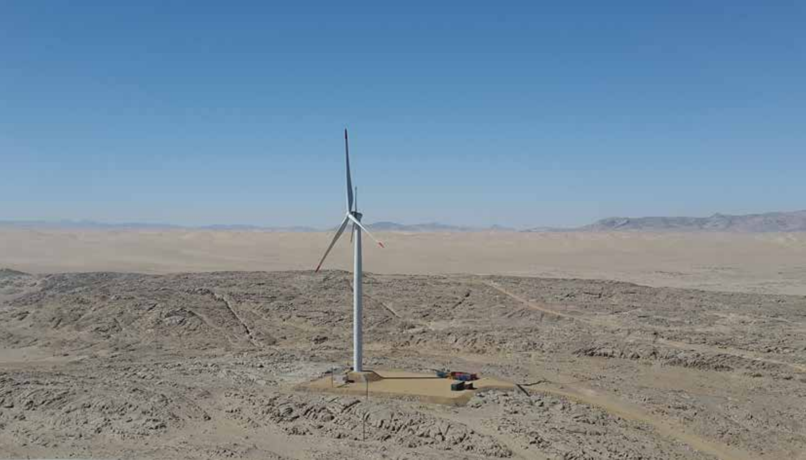
Ombepo Energy is Namibia's first wind farm and it was financed by DBN
