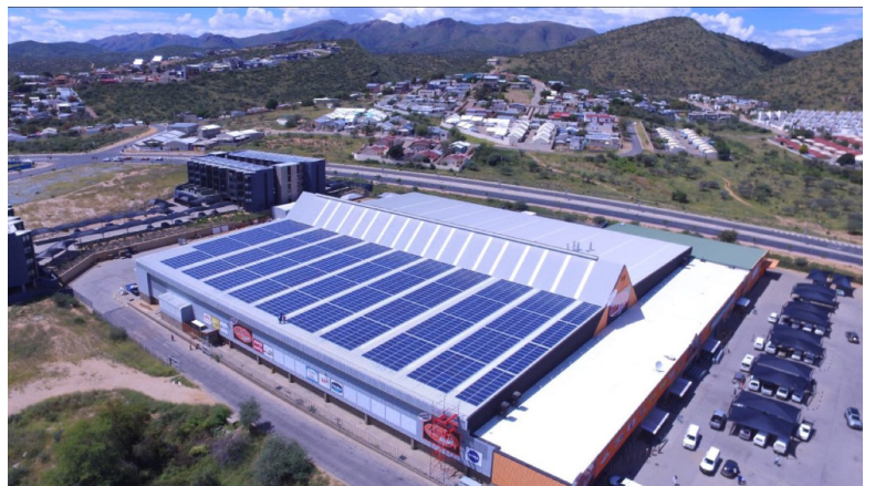
The Metro Hyper rooftop in Kleine Kuppe is adorned with solar panels from Solar Saver
