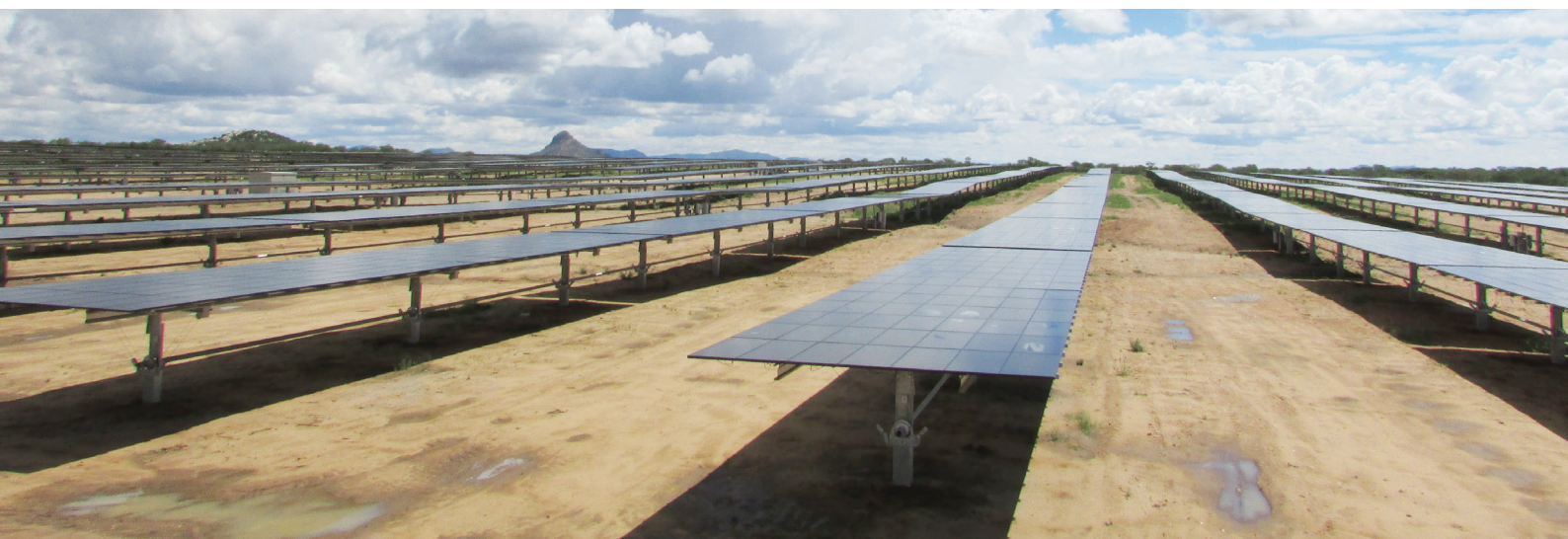
PIONEERING PROJECT: The Omburu solar plant near Omaruru constructed by InnoSun energy with support from the DBN
