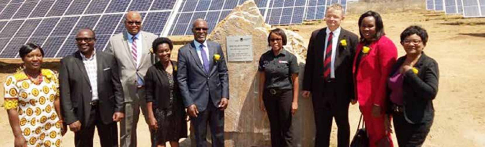
The recently-inaugurated 5 megawatt Sun EQ solar facility at Otavi which was financed by DBN
