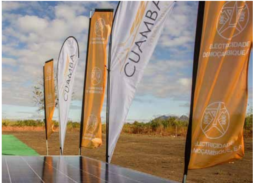
Globeleq and project partners, Source Energia and Electricidade de Moçambique (EDM), have started constructing a solar PV plant with energy storage in Cuamba, Mozambique
