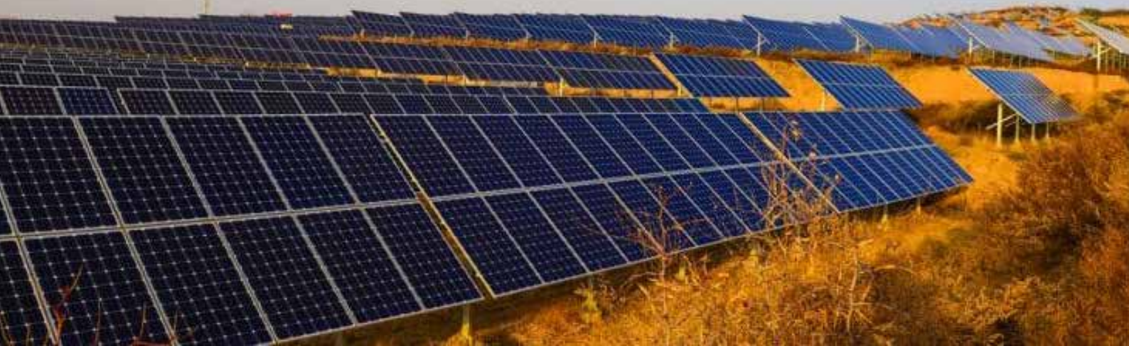
The Omburu plant, located adjacent to the NamPower transmission station some 12km from the town of Omaruru, is being constructed by the joint venture of Hopsol Africa and Tulive Private Equity on behalf of NamPower
