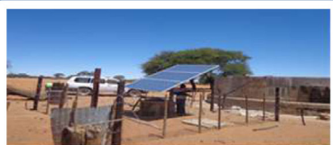
A Photovoltaic Pumping System produces energy for pumping water for livestock and domestic use.
