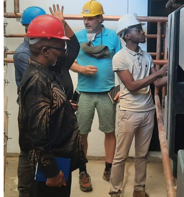
INSPECTION ... Engineers from the SOLTRAIN project and NEI inspecting the Lady Pohamba Private Hospital installation.
