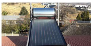
A Solar Water Heater uses energy from the sun to heat water for domestic use.
