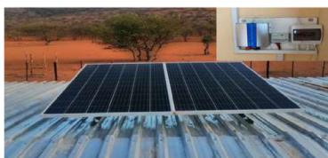
A Solar Home System typically has the capacity to power lights and devices such as radios, TVs, fridges and cell phone chargers.
