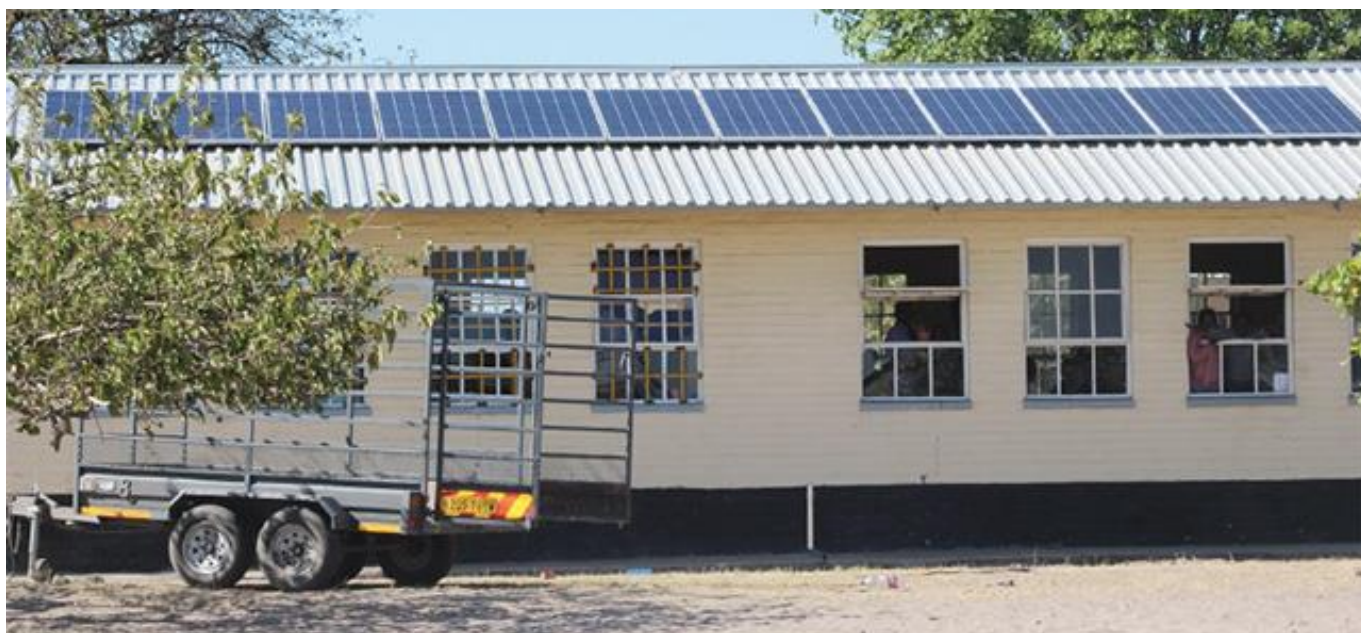
CLASSROOM SOLAR: Installed Solar panels at Nsundwa Combined School in the Zambezi Region
