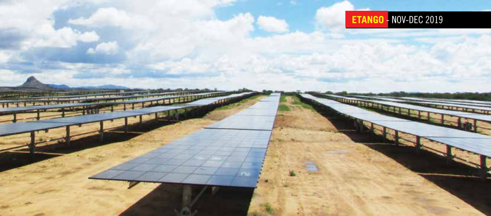
Omburu is currently home to this 4.5MW solar plant developed by InnoSun in 2015
