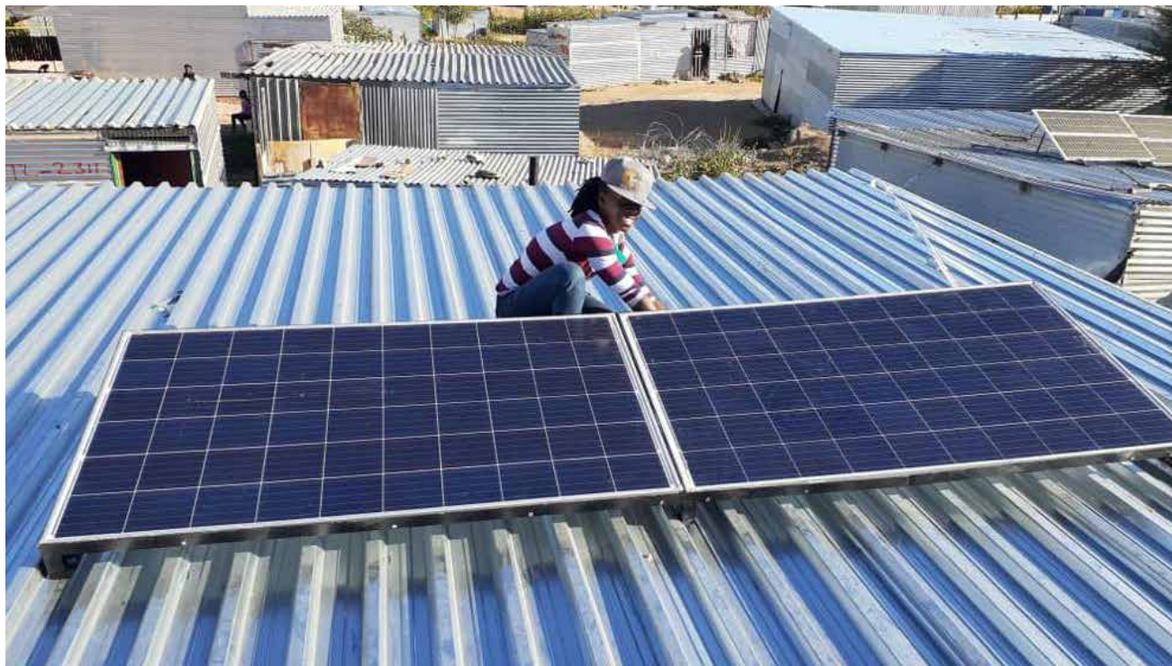
INSTALLATION ... Charity Thebuho Taatisolar PV engineer on the roof inspecting a solar installation.
