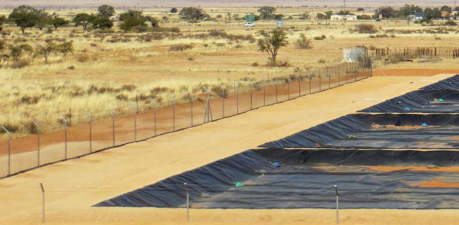
The Pilot Groundwater Desalination Plant at Grünau, in the //Karas Region
