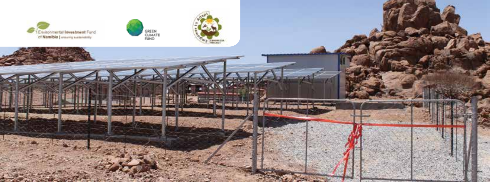
The 150-kilowatt solar plant erected at the Soris Soris Conservancy
