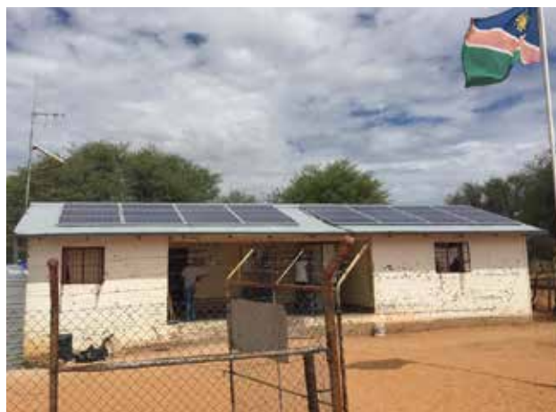
SOLAR-POWERED CLINIC: Installation of solar energy photovoltaic (PV) systems at remote clinics will improve access to quality health services in Namibia
