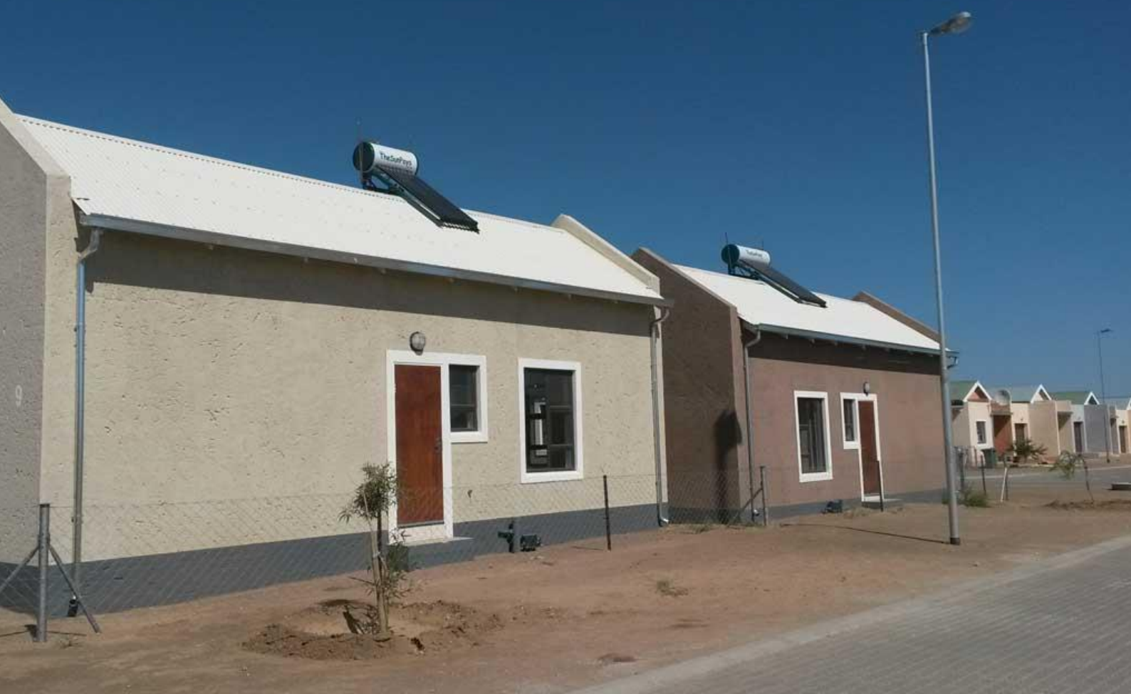
Some of the solar water heating systems that were built in the Osona Village Project in Okahandja
