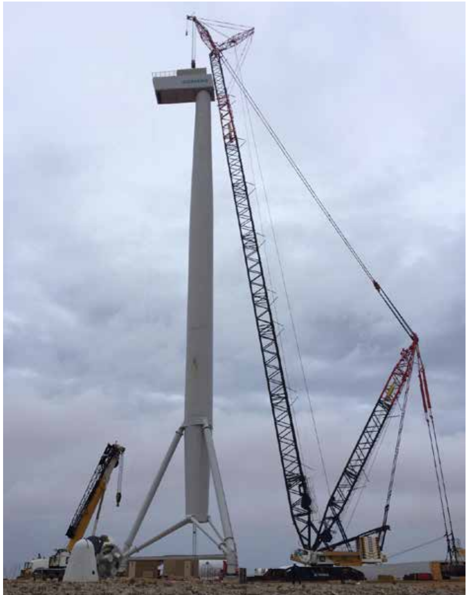
An installation of Nabrawind's Nabralift Tower at the Oualidia project in Morocco. The project is run by InnoVent, InnoSun's parent company
