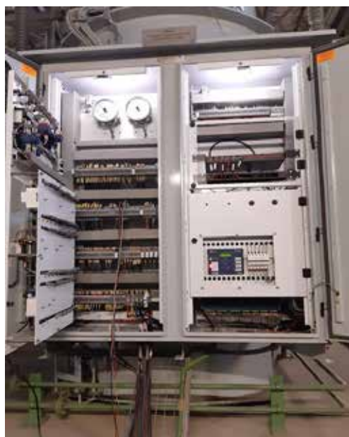
NEW... The new installation
