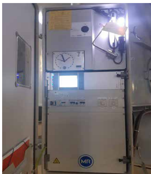
OLD... The old installations which were malfunctioning and failing that have now been replaced.
