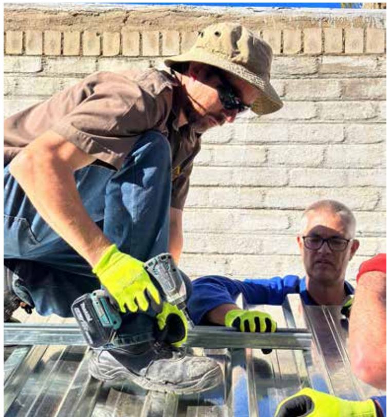
NEW SKILLS ... Learning to attach mounting structure on IBR training roof. -GREEN Solar Academy
