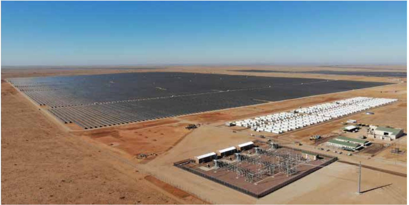
MEGA PROJECT ... The Kenhardt project is one of the world's first and largest hybrid solar and battery storage facilities, with an installed solar capacity of 540MW and a battery storage capacity of 225MW/1,140MWh. Photo: Scatec
