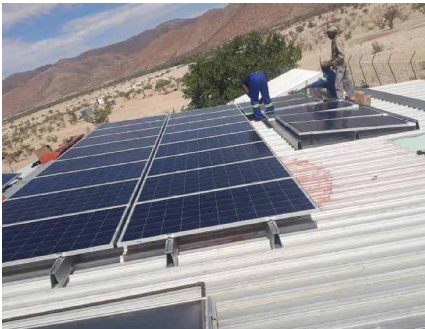
RURAL SUPPORT: Through the Solar for Health Project, solar panels were installed in rural clinics across Otjozondjupa, Kavango East, and Kunene—supporting the Ministry of Health and Social Services to improve patient care and reduce energy costs.
